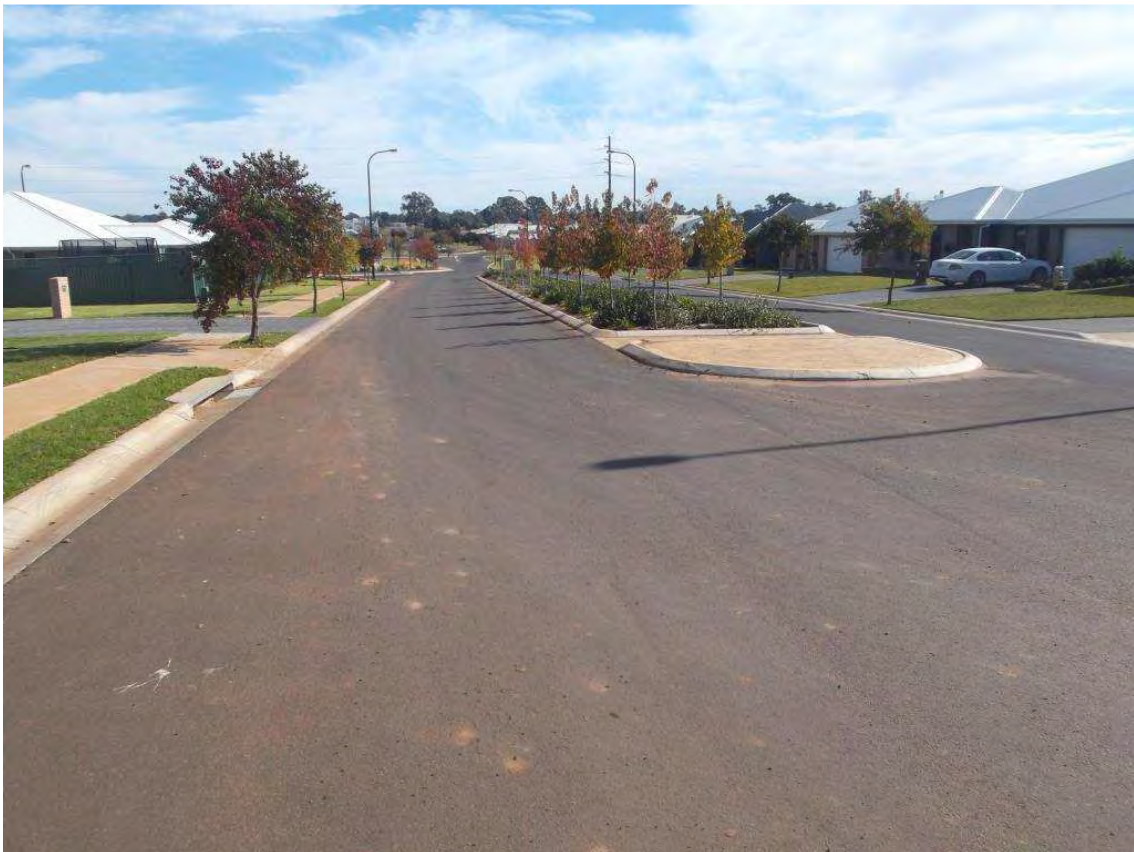
Plate 20: Typical road carriageway in Azure Avenue
