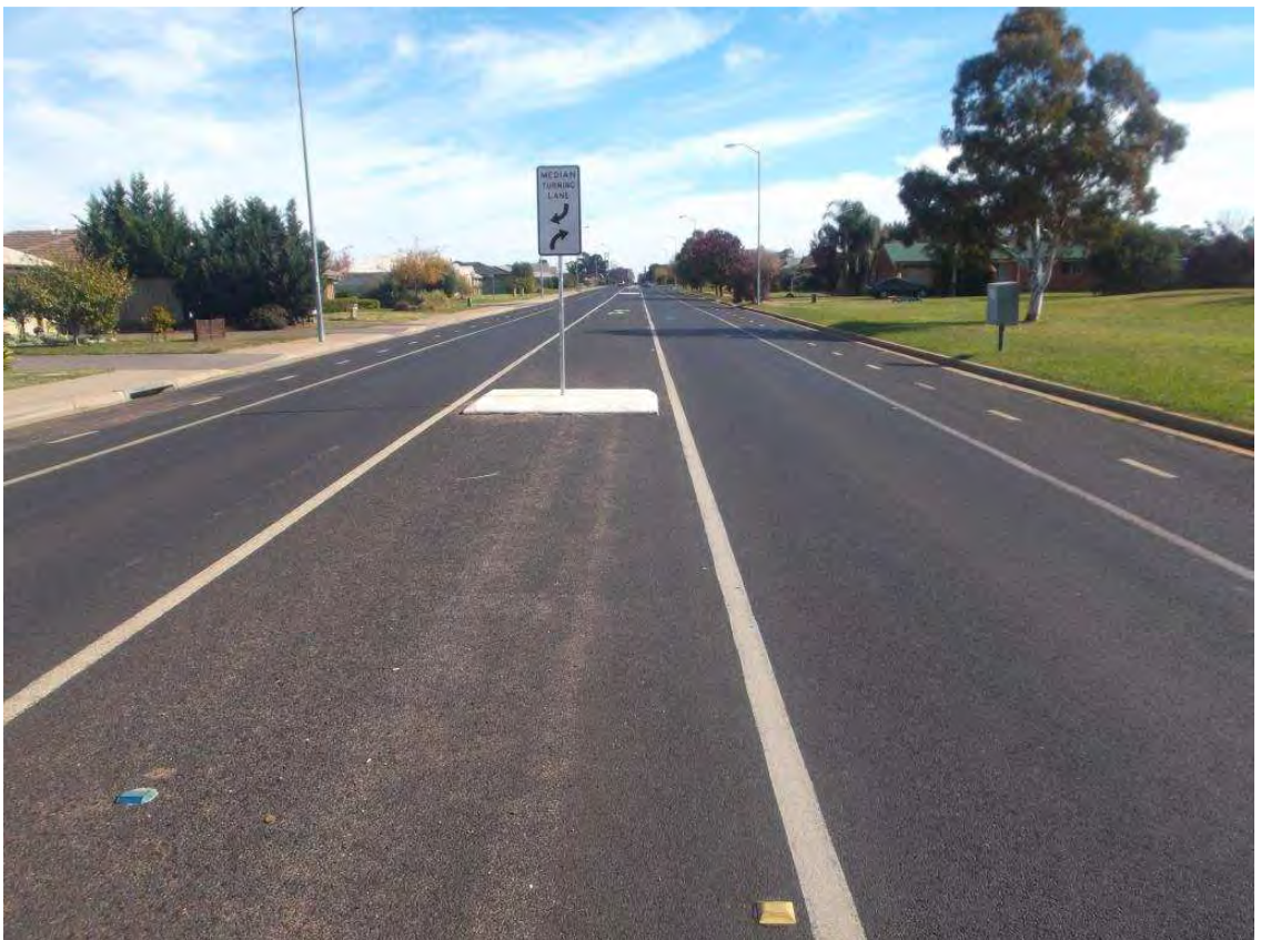
Plate 4: Boundary Road westbound
