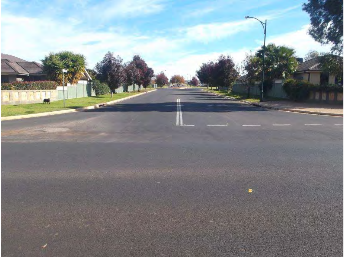
Plate 11: Intersection of Wheelers Lane and Holmwood Drive
