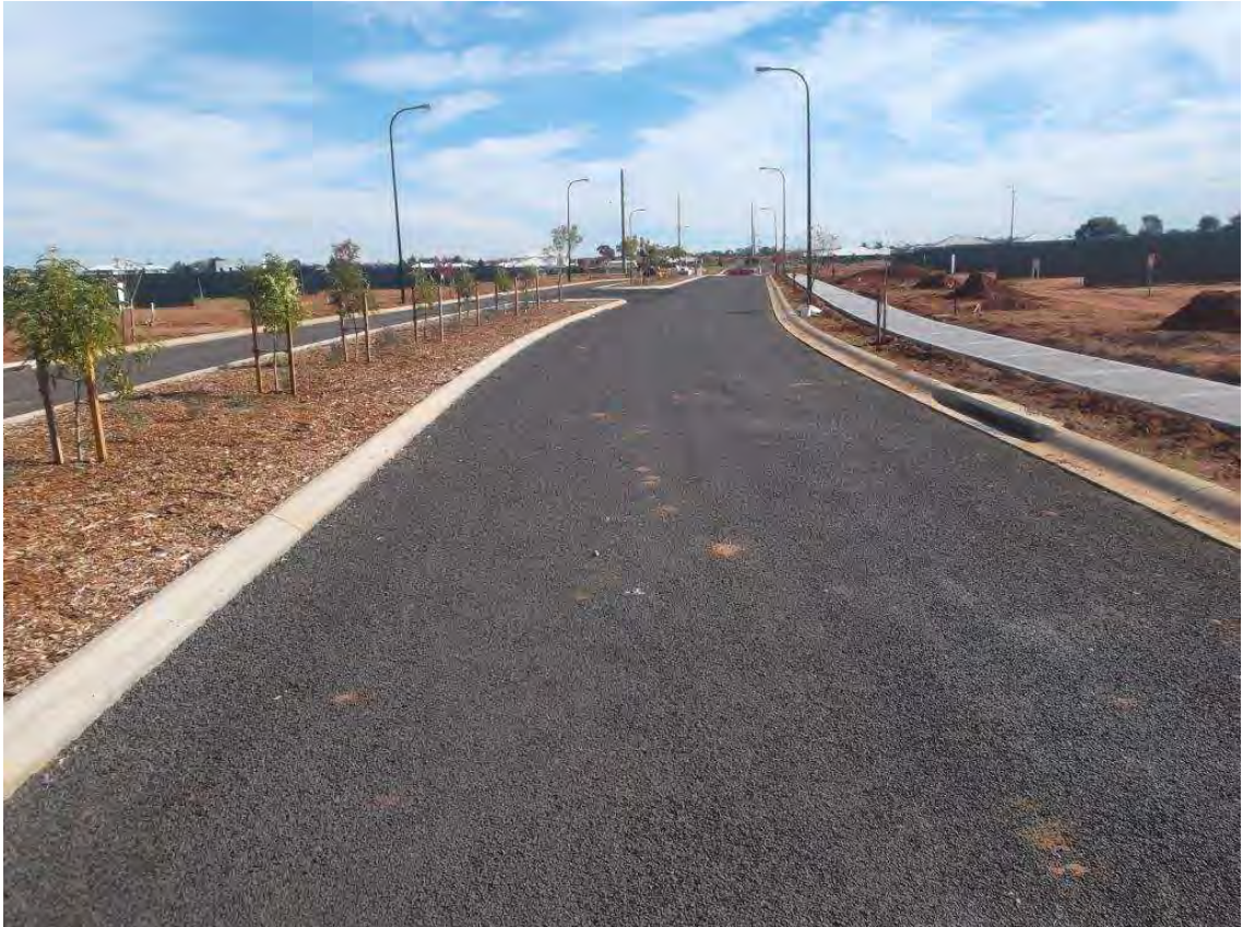
Plate 21: Typical road carriageway in Argyle Avenue
